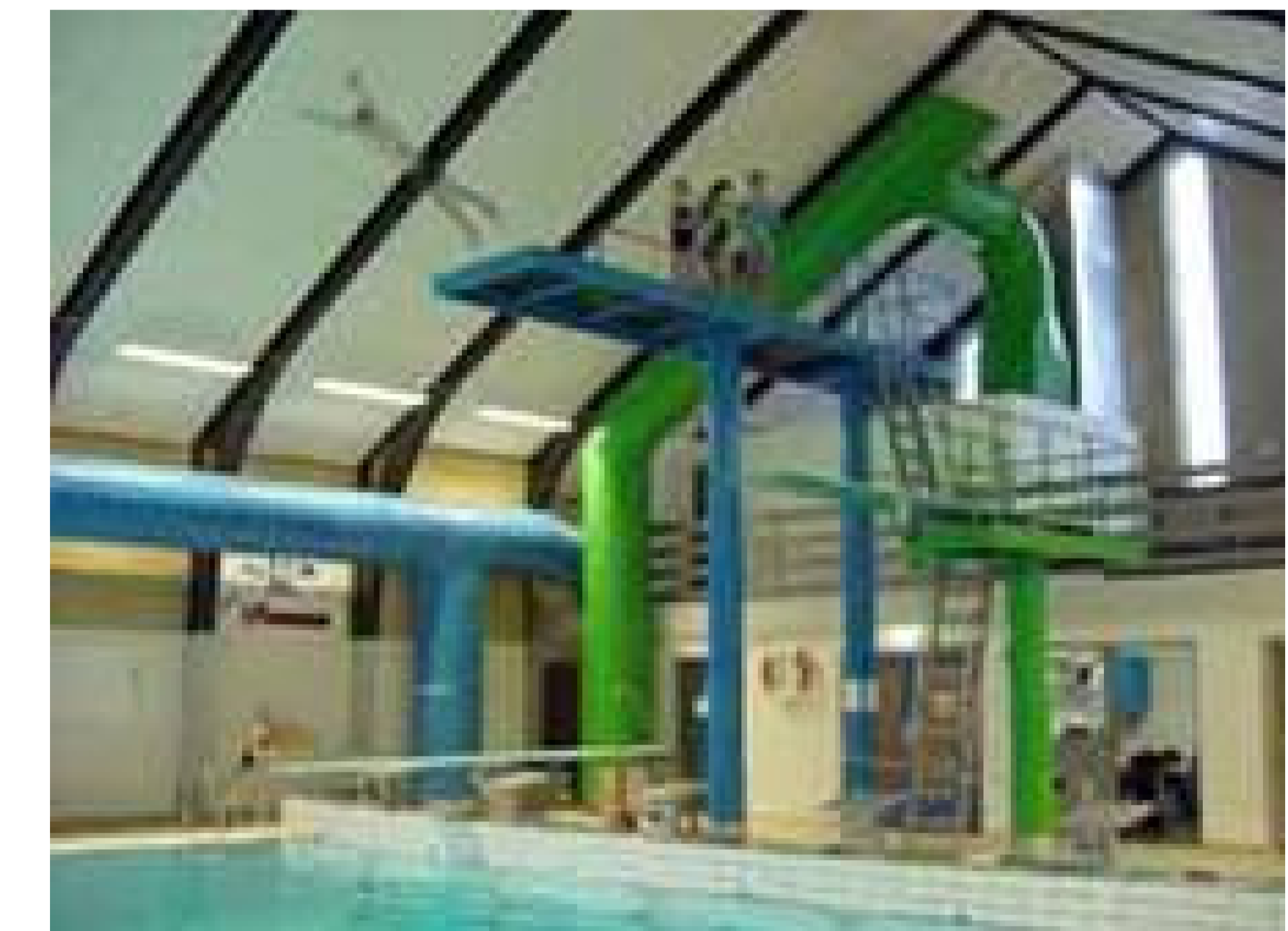
The swimming hall has just been renovated
