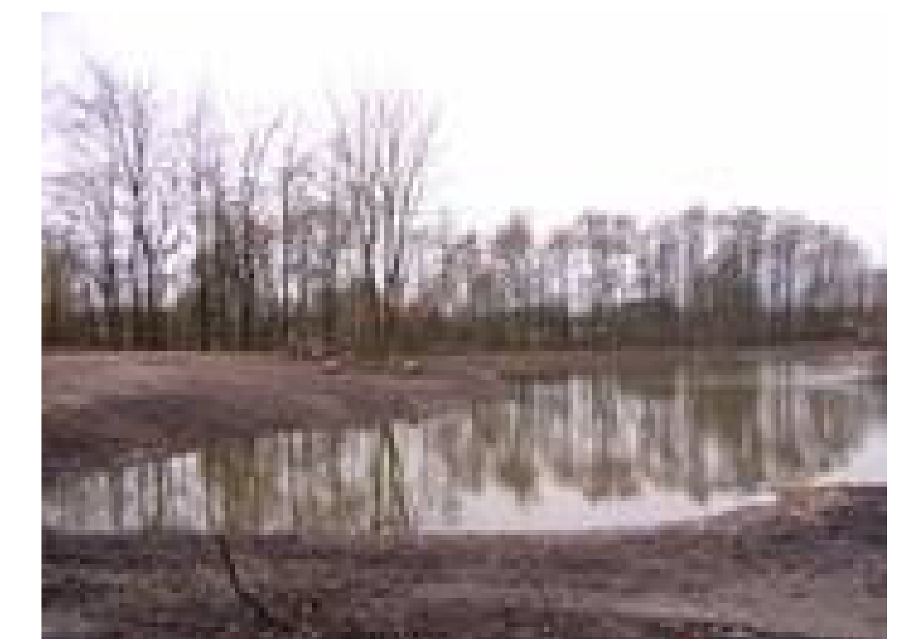
The lake is taking form in the new village park
