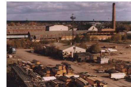
The industrial area (backyard)
